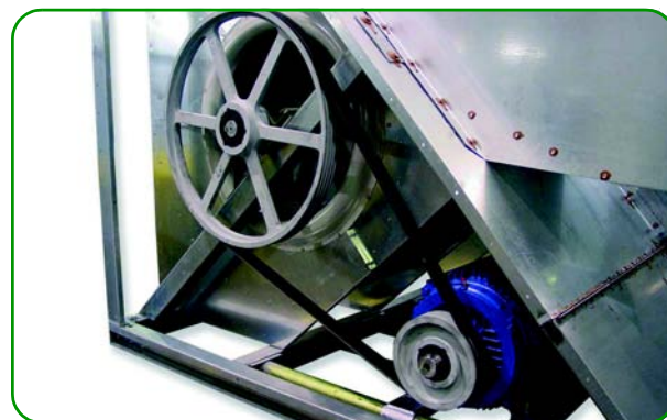
External V-belt drive system (shown here with panel removed)
